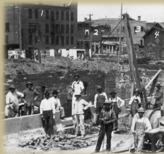
Moscow federal building under construction. (University of Idaho)
