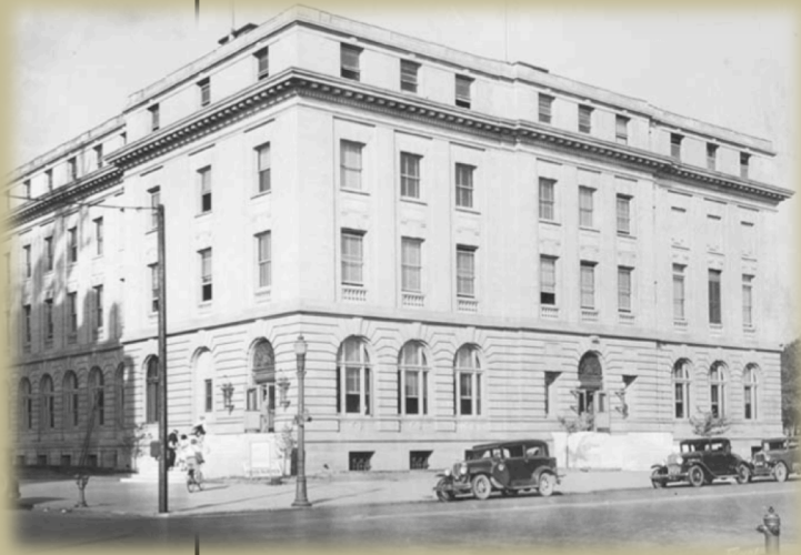
Federal courthouse at Boise, 1905. (Idaho State Historical Society)
